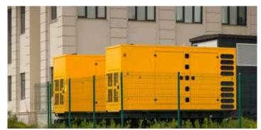
centers delay starting generators for a few seconds after utility power failure. Including this delay, generator starting and providing power to the UPS and other loads is typically complete in less than 30 seconds. Installations with large arrays of parallel generators and less-than-optimal generator paralleling controls may require up to one minute.
